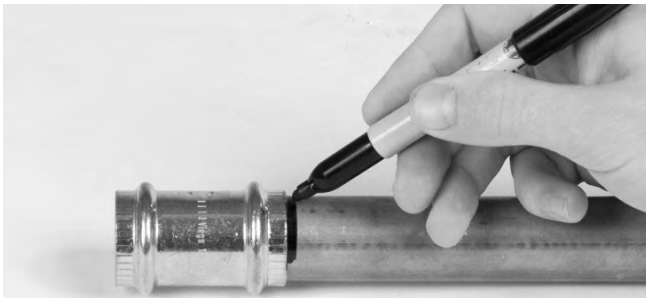
Figure 8 – Marking the Tubing After Fully Inserting Tube
