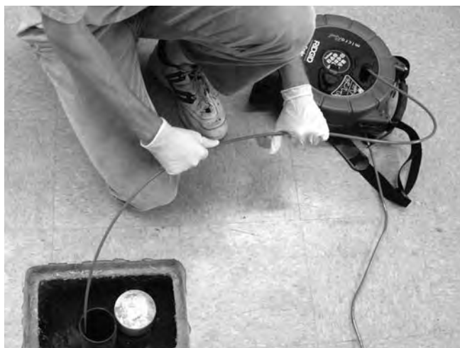
Figure 29 – Allowing cable to loop may kink the cable while pushing into drum
