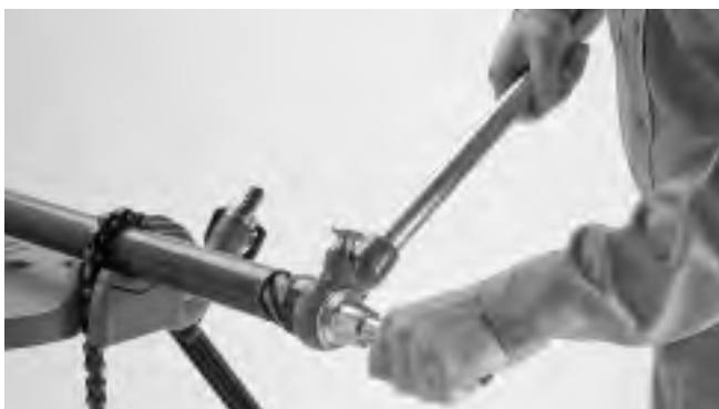
Figure 2 – Reaming End of Pipe
