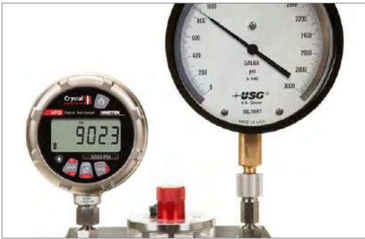
Checking the accuracy of an analog pressure gauge against the display of the reference.
