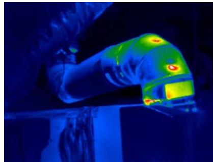
INSPECT DUCTS AND VENTILATION
