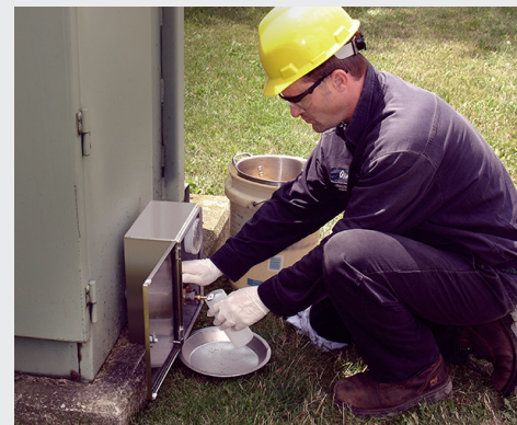
External Oil Sampling – Courtesy of SDMyers
